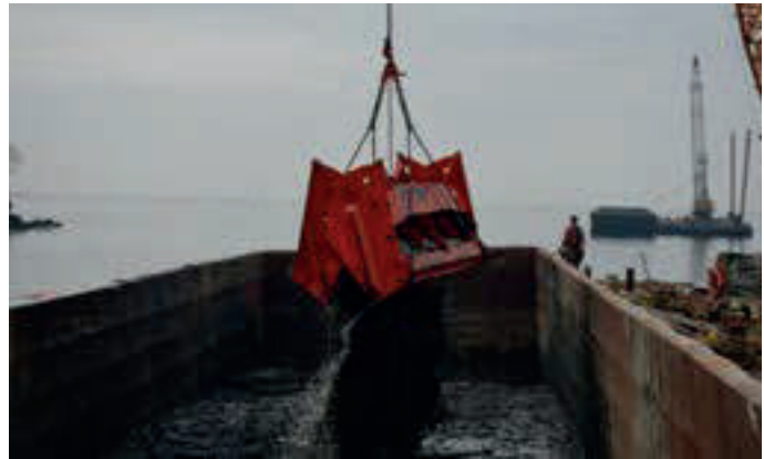
Clamshell bucket placing dredged material into scow
